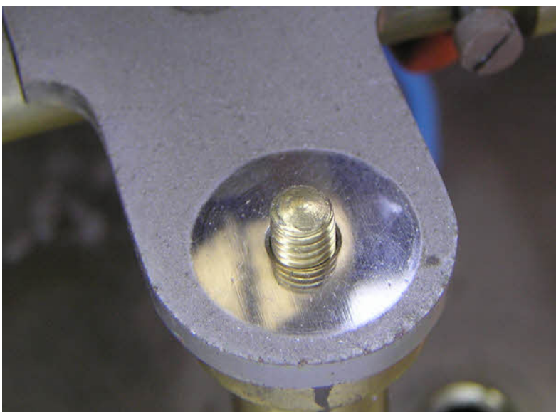
The condition of the nickel plating under the ornate finial nuts is in almost perfect condition compared to the unprotected areas.
