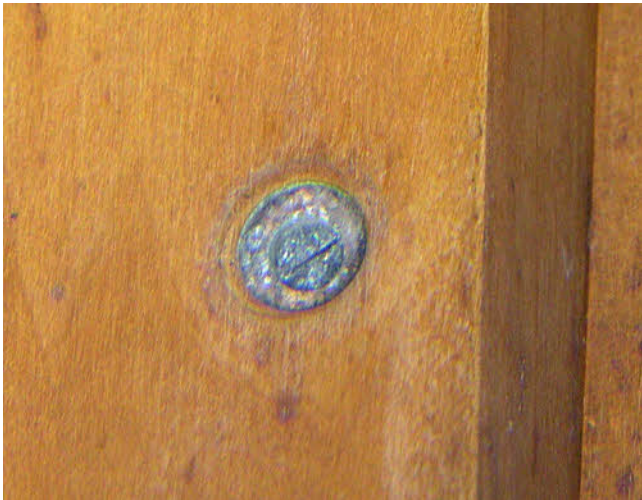
The corroded pillar securing screw from the rear.
